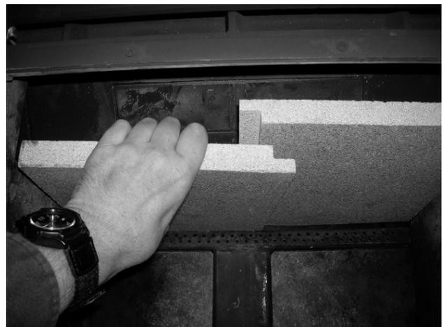
Figure 16 - Removing/Replacing the Baffle for Inspection
